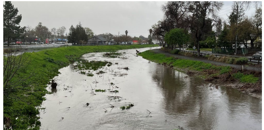
The capacity of Grayson Creek in Pacheco has been increased to protect against flooding
