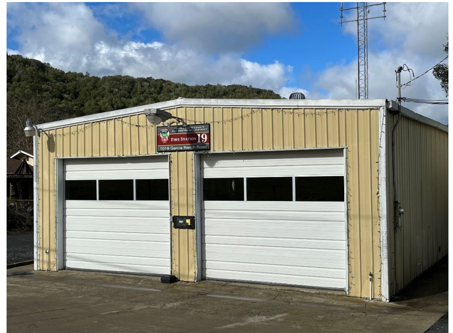
The Contra Costa Fire Protection District operates this station in rural Briones Valley.
