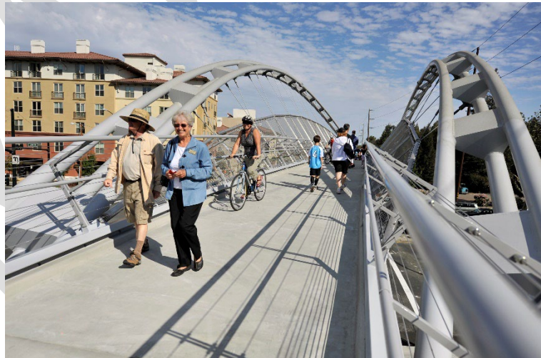
Contra Costa Centre Overcrossing
