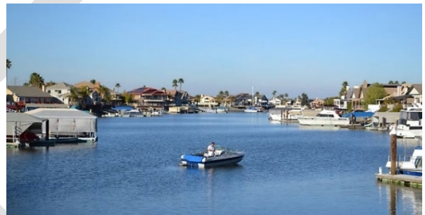
Sea level rise and other coastal flooding hazards threaten structures built near the shoreline.
