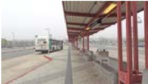
The Pittsburg/Bay Point BART Station.
