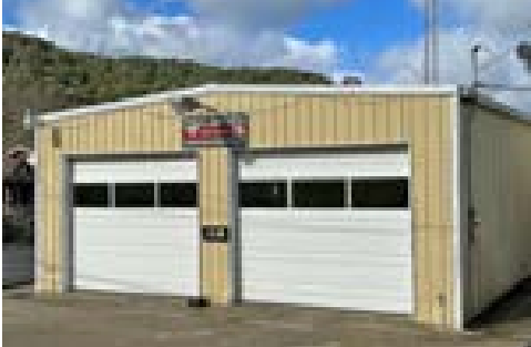
Existing fire station in Briones.
