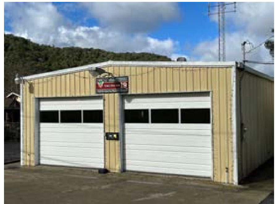
The Contra Costa Fire Protection District operates this station in rural Briones Valley.
