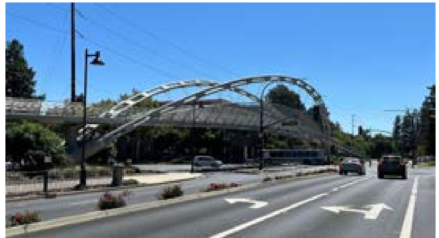
The Robert I. Schroder Overcrossing along the Iron Horse Trail is part of an important non-motorized regional connection between Pleasanton and Concord.
