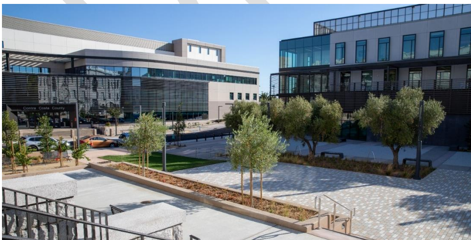
The new Contra Costa County Administration Building, part of the first government project in the world to receive TRUE pre-certification. Photo credit: Contra Costa County staff.
