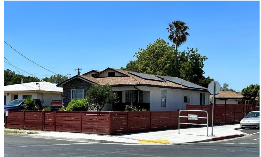
Solar panels help reduce reliance on natural gas and electricity providers and increase resilience for homeowners.
