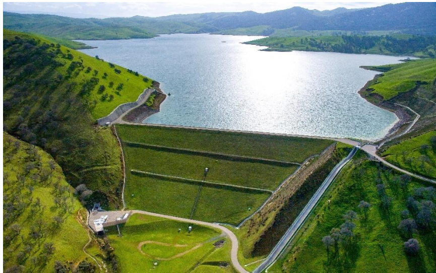
Los Vaqueros Reservoir is integral to the county's water supply.
