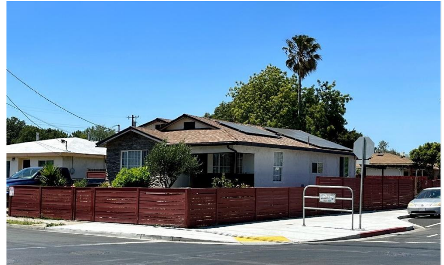
Solar panels help reduce reliance on natural gas and electricity providers and increase resilience for homeowners.
