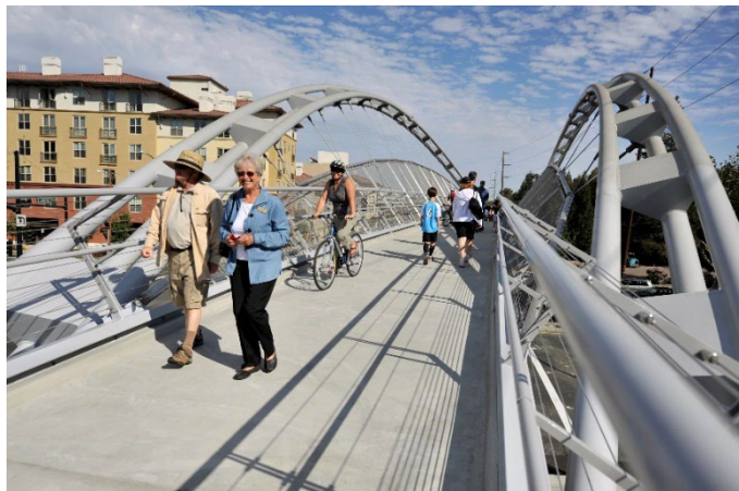
Contra Costa Centre Overcrossing. Photo credit: Contra Costa County
