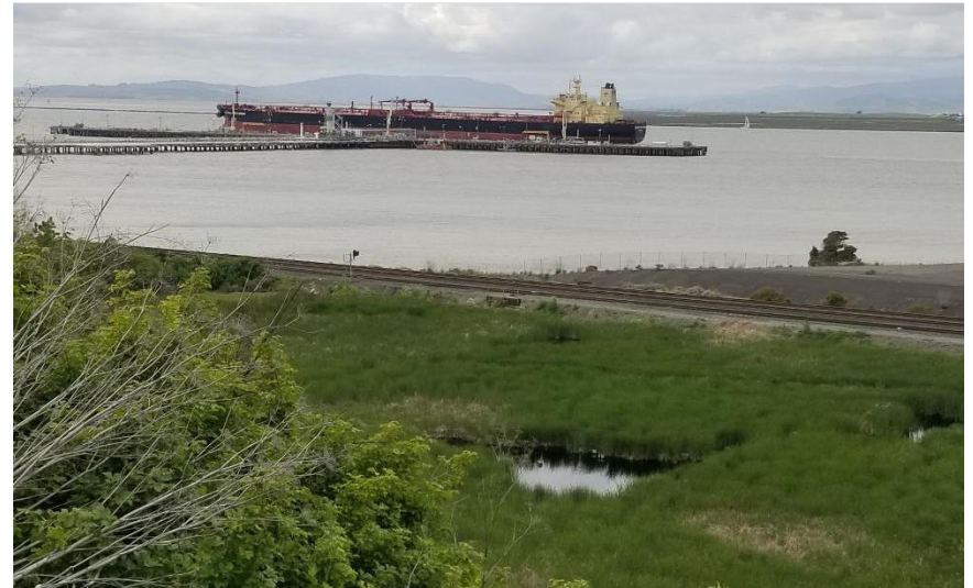
Contra Costa County is part of the global shipping economy through various local ports, marine terminals, and railroads.
