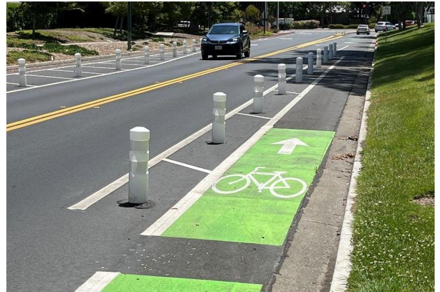
Separated and protected bicycle facilities increase the usage and safety of bicycles as a mode of transport, helping to shift trips away from automobiles.
