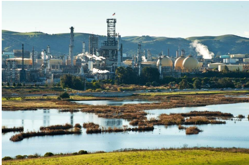
Emissions from heavy industrial facilities disproportionately affect Impacted Communities. (Credit: California Department of Water Resources)
