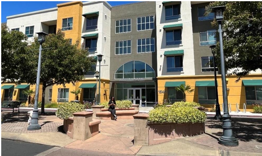
Streetscape improvements like this project along Fred Jackson Way in North Richmond are provided by the County's Public Works Department.
