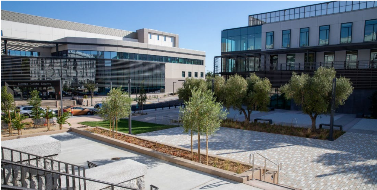
The new Contra Costa County Administration Building, part of the first government project in the world to receive TRUE pre-certification. Photo credit: Contra Costa County staff.
