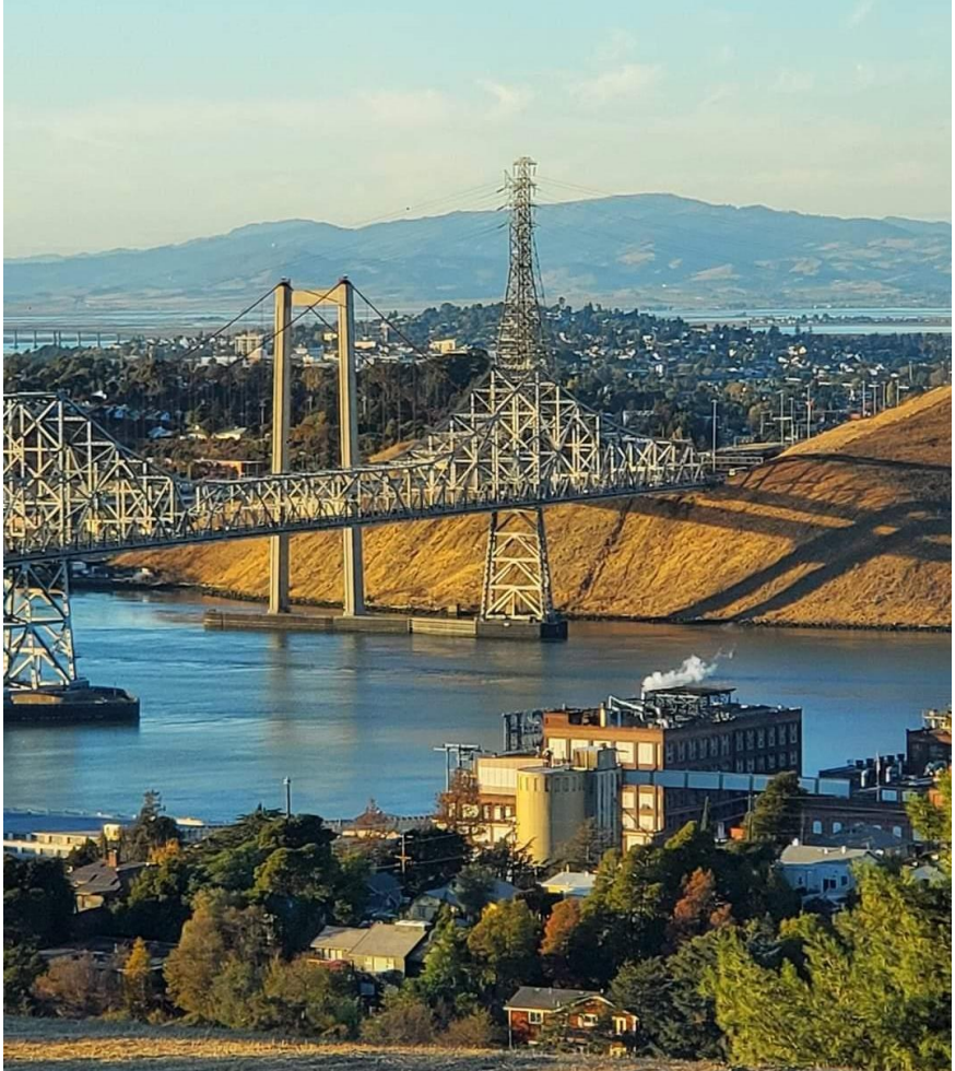
The historic C&H Sugar Refinery provides local jobs and bolsters the Crockett economy. (Community-submitted photo)
