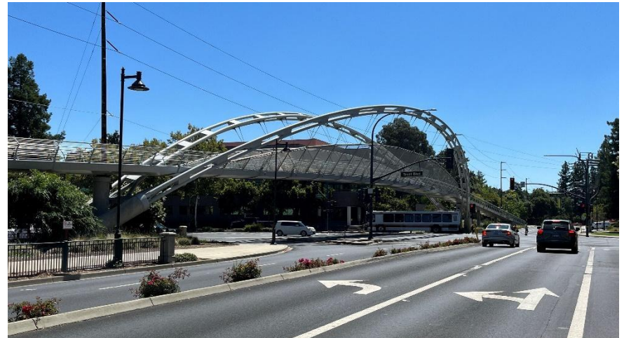
The Robert I. Schroder Overcrossing along the Iron Horse Trail is part of an important non-motorized regional connection between Pleasanton and Concord.
